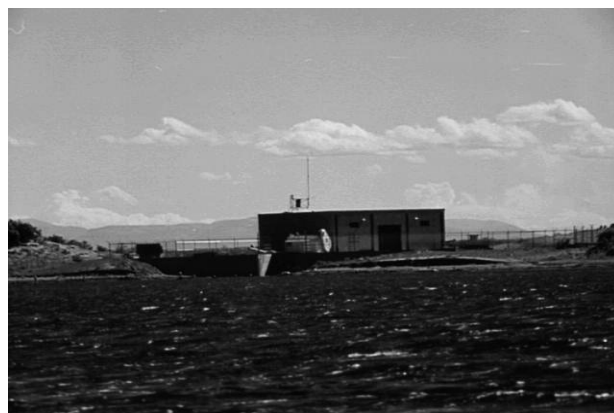
Figure 4 San Luis Lake Pumping Plant
