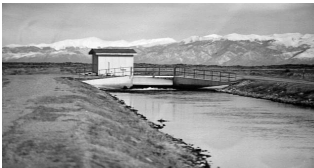
Figure 3 View of Parshall Flume & Conveyance Channel
